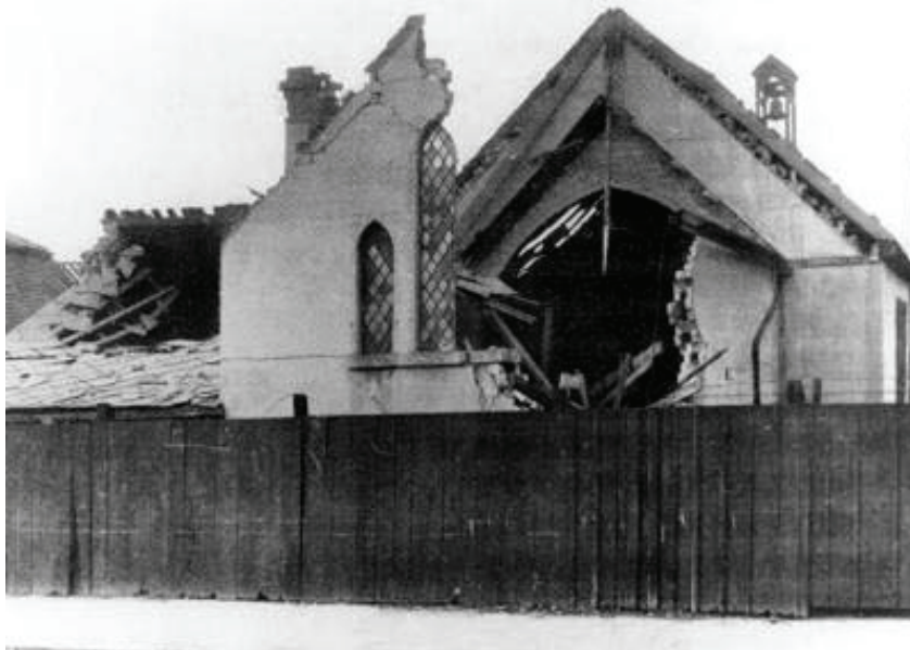
Damage to St. Barnabas Church Westwood Road
