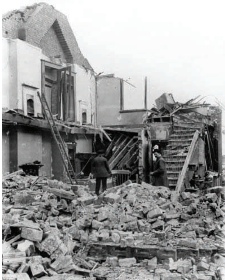
Houses damaged in the Silvertown Explosion January 1917
